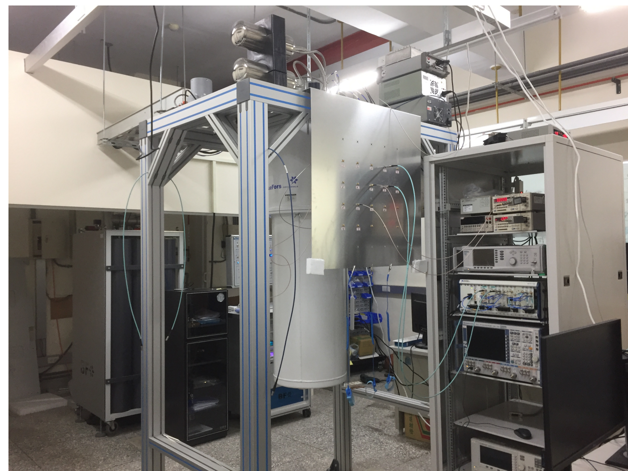
Max 50 Coax cables
